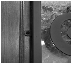
Photo 1: standard mount of iron grille
